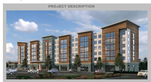
The facility is a new, 120-room Residence Inn by Marriott extended stay all-suites hotel with a one-story natatorium annex. The hotel structure is a pile-supported ground-floor structural slab; elevated floors are reinforced lightweight concrete slabs on composite decks supported on loadbearing metal studs. Ground floor public area is supported by structural steel framing system, the natatorium is supported by structural steel-framed walls with glue-laminated timber beams supporting the roof.
